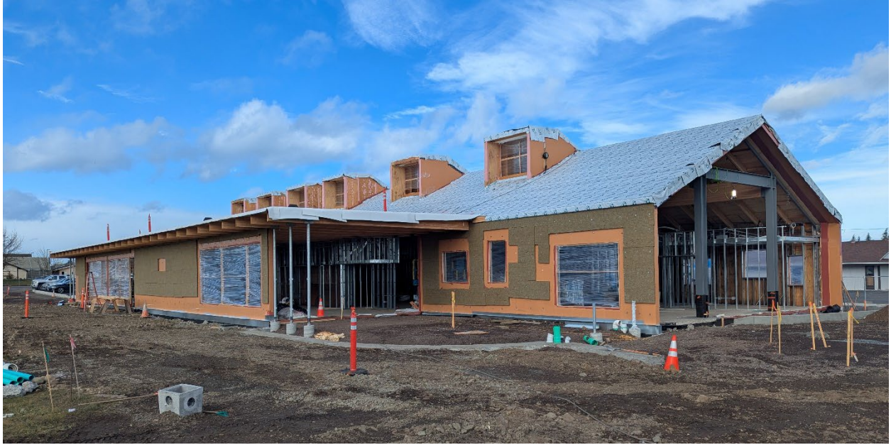
The Sequim Library under construction in March 2025.
