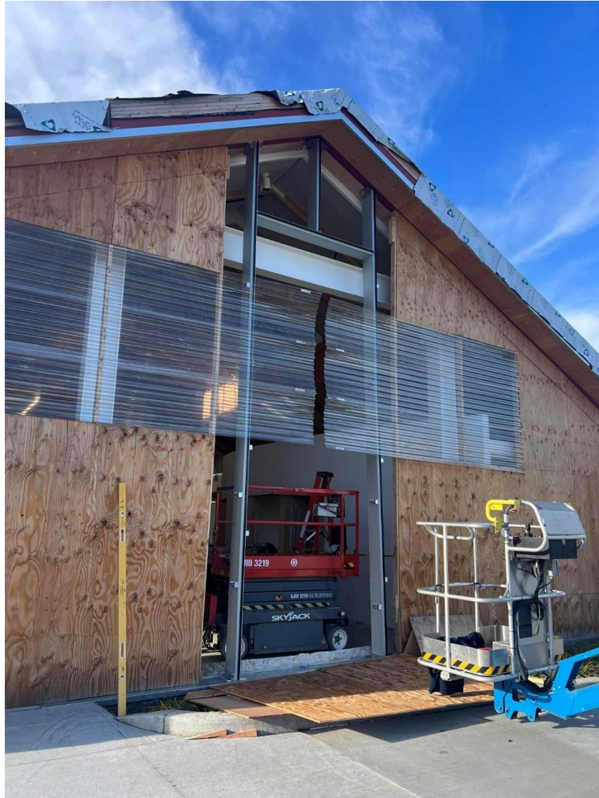
Temporary wall materials are being removed to allow for the installation of framing and windows on the east wall of the Sequim Library on December 22, following the arrival of specially fabricated materials.
